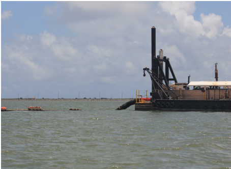
Dredge operating near Galveston Island. (Photo Credit: Texas General Land Office)
