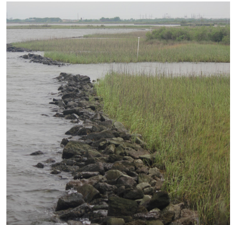
Living shorelines along the Texas City Prairie Preserve at Moses Lake. (Photo Credit: Texas General Land Office)
