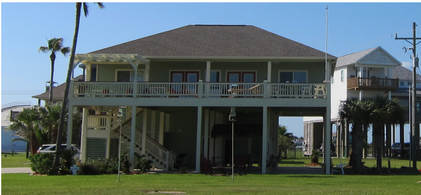
An example of an elevated home on Bolivar Peninsula. (Photo Credit: Texas General Land Office)
