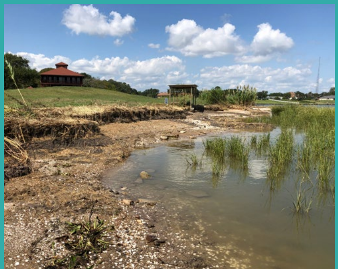
Erosion along Trinity Bay (Photo Credit: Galveston Bay Foundation)
