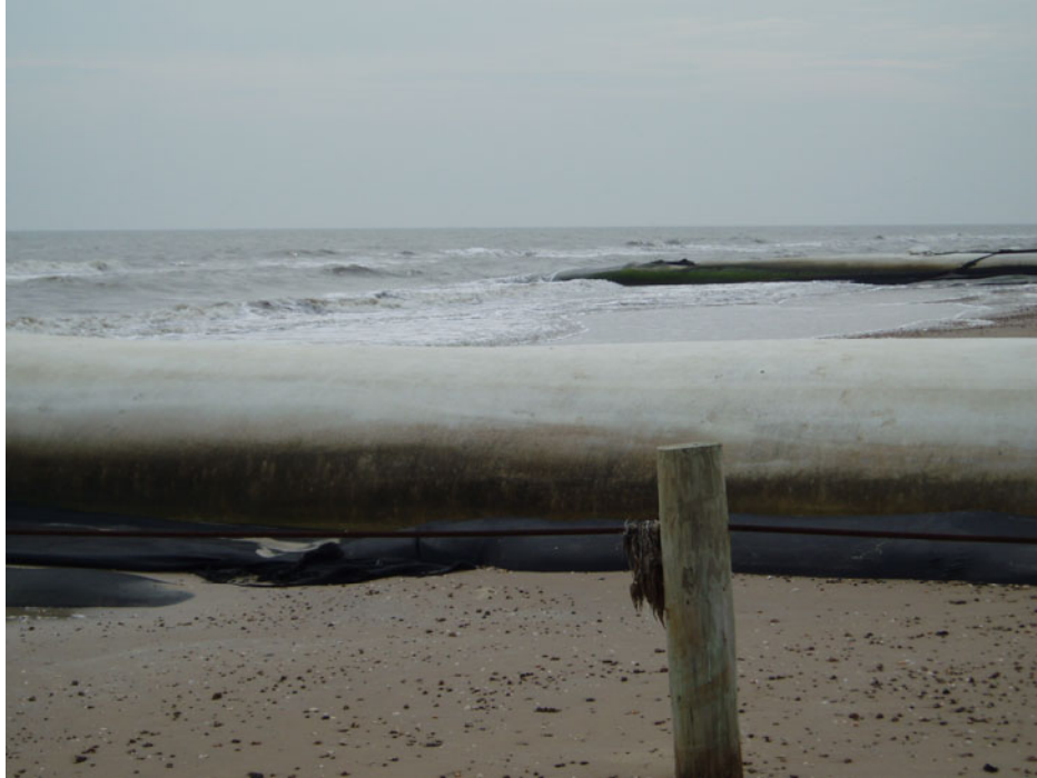
Figure 8. Geotubes placed along the Gulf shoreline on the McFaddin NWR to help trap sediments and slow shoreline erosion show up well on Lidar images. See previous Lidar figure for plan view of tubes. Above photograph was taken from the northeast end of the tube field.
