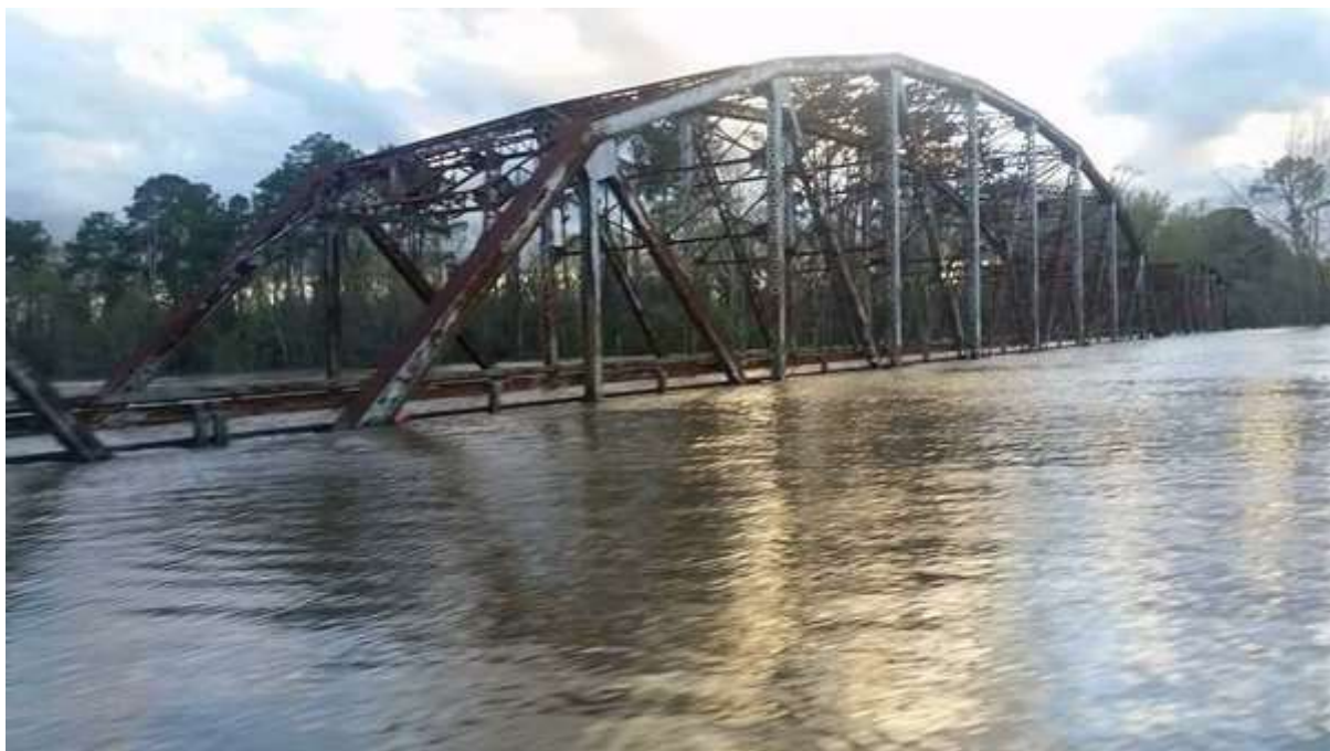
Burr’s Ferry Bridge SH 63 over Sabine River – photo by Texas Department of Transportation
