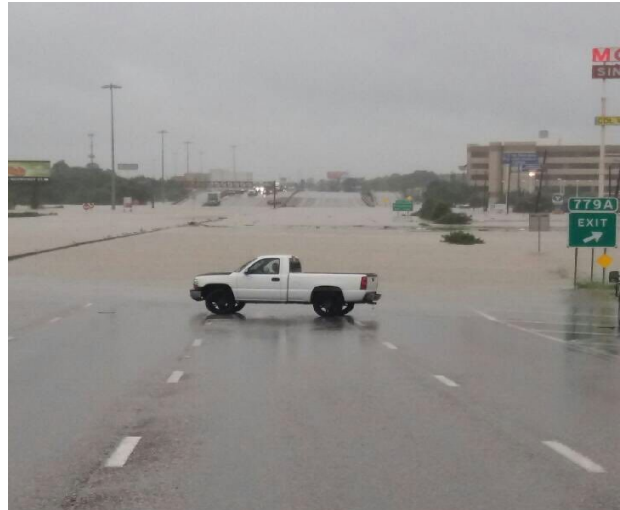
Source: HOU District Twitter feed – Aug 28, 2017 ( https://twitter.com/TxDOTHoustonPIO )
