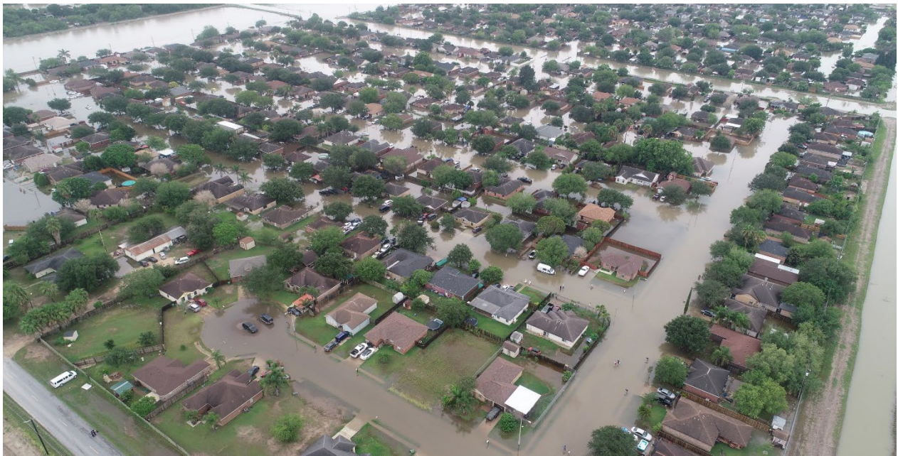
Figure 2-1: Flooding in Hidalgo County (Weslaco, Texas) 12
