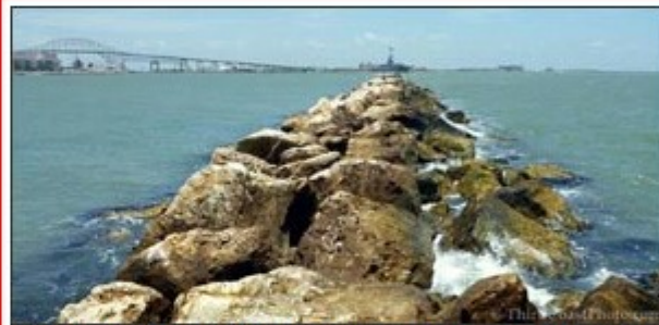
A breakwater could solve the recurring problem of erosion on North Beach.
