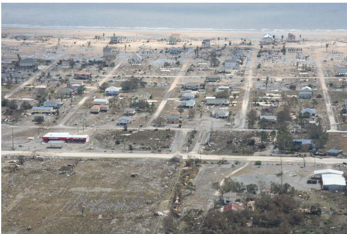
Figure 3-27: Bolivar Peninsula, Texas, after Hurricane Ike. 70
