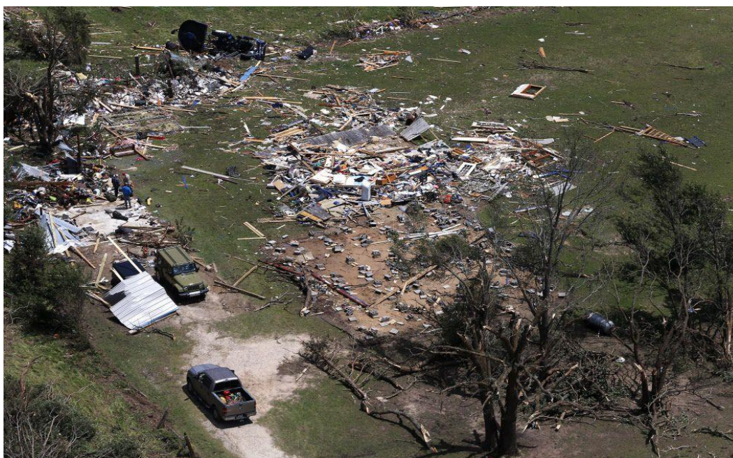
Figure 3-49: Destroyed home in Canton, April 2017 tornadoes. 237
