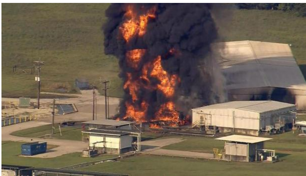
Figure 3-67: Arkema chemical plant explosion in Crosby in 2017. 404
