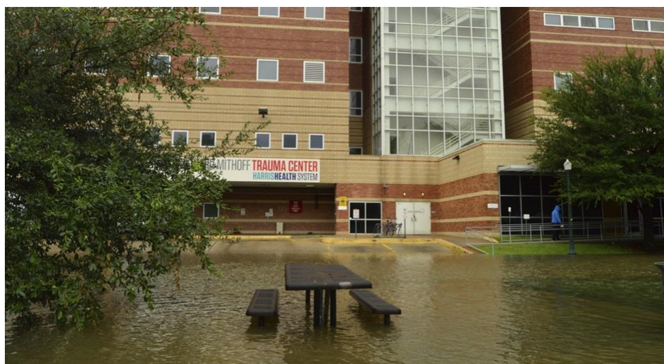
Figure 3-31: Hurricane Harvey floodwaters approach Ben Taub Hospital in Houston. 115
