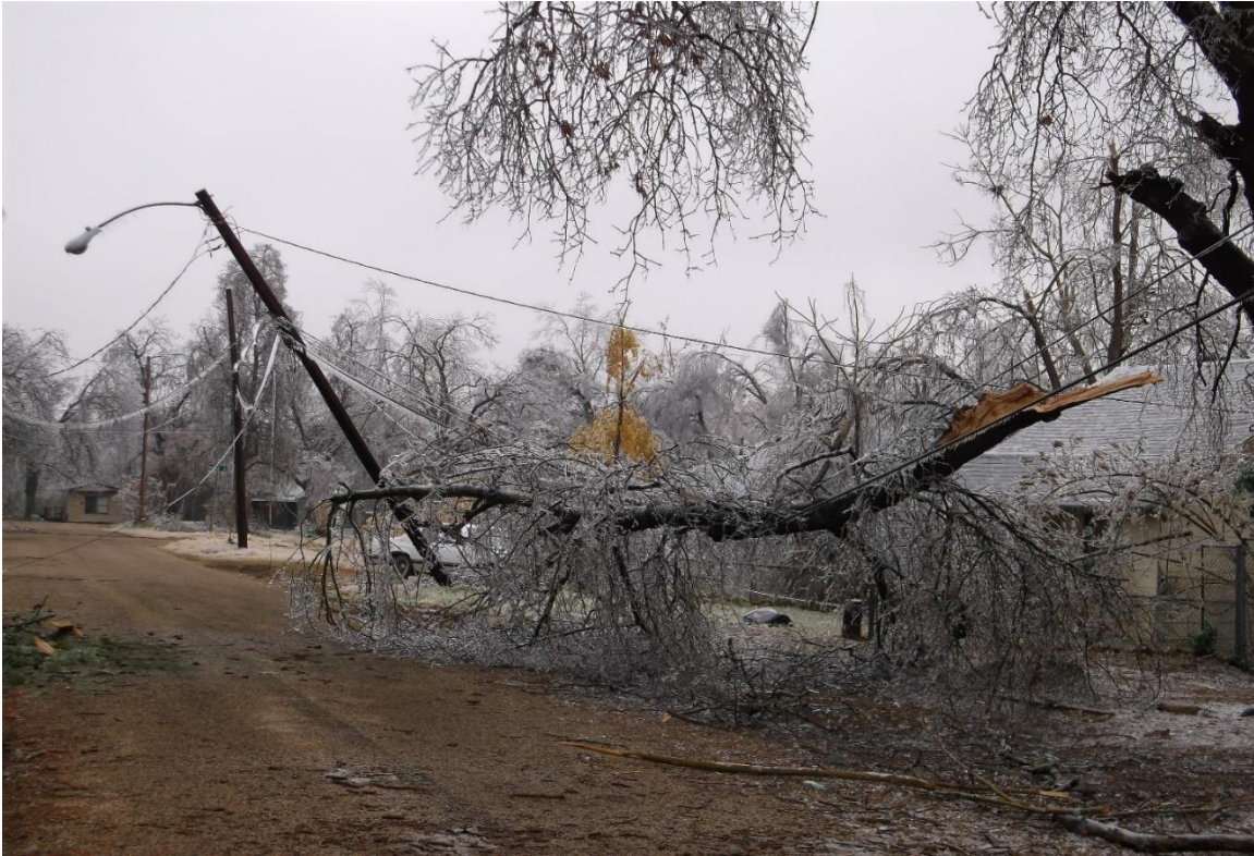
Figure 3-60: Downed power line during the 2013 ice storm in Paris, Texas. 334
