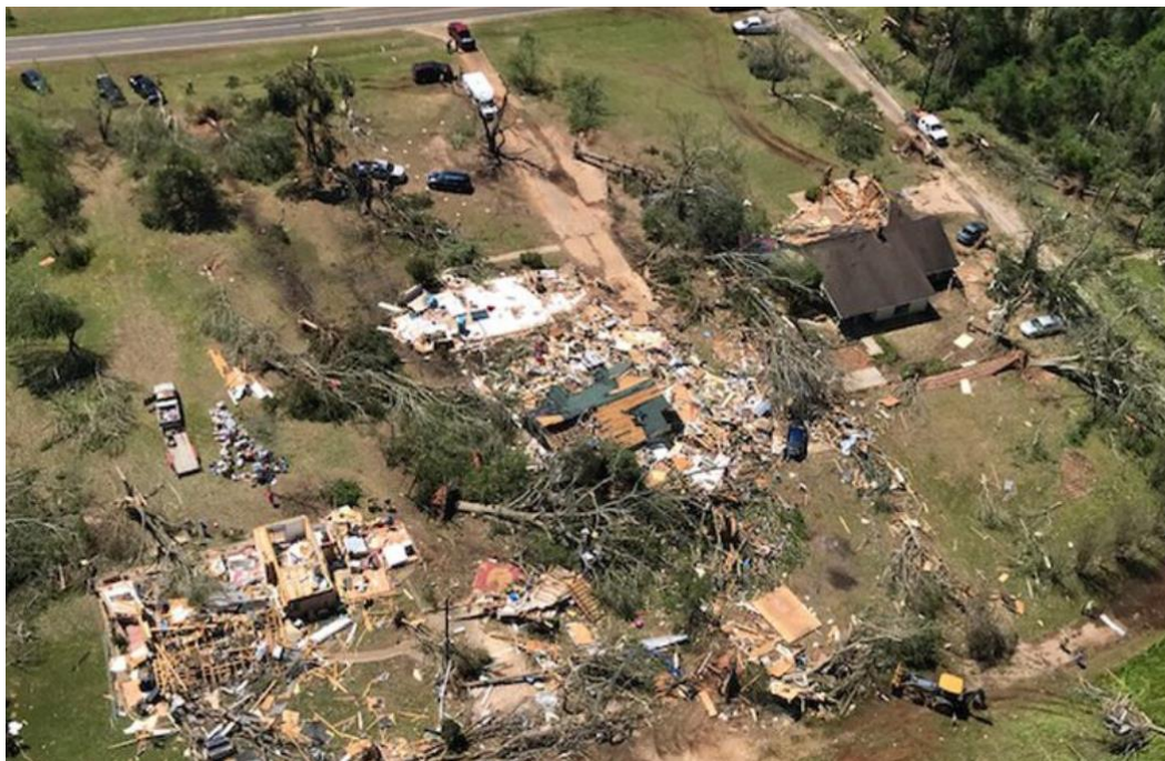
Figure 3-48: Residential tornado damage in Cherokee County, April 2019 tornadoes. 234
