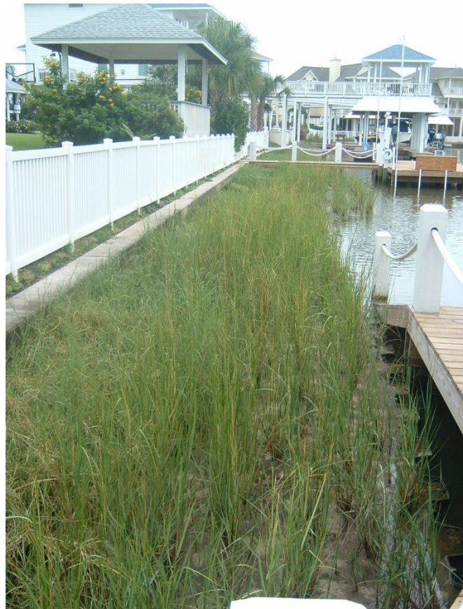
Figure 3. Landowner Living Shoreline in Laffite's Cove, Galveston. Photo Courtesy of Galveston Bay Foundation.
