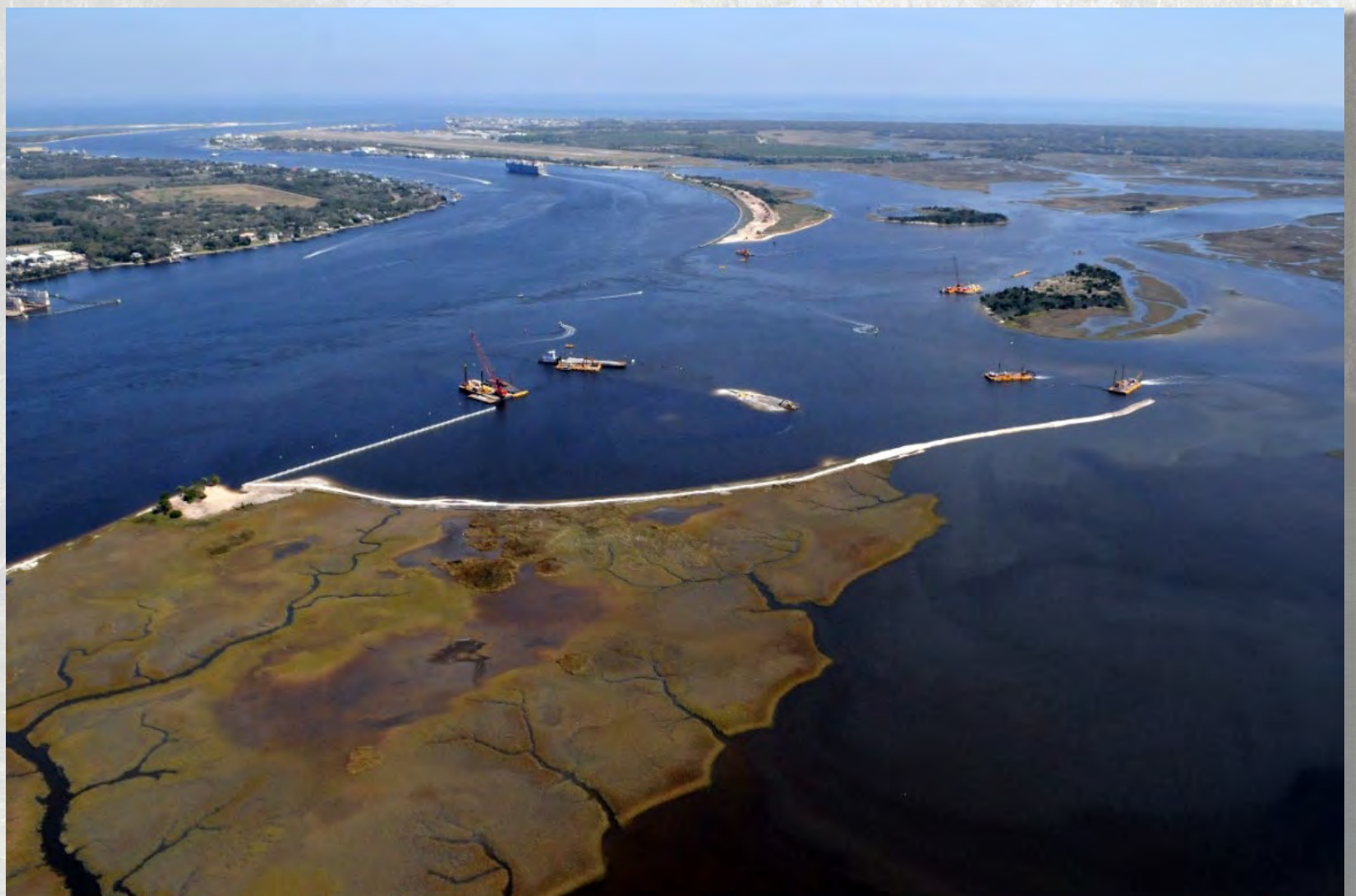
Great Marsh Island, Jacksonville, Florida [Infrastructure Alternatives, Inc. / Manson Construction Company]
