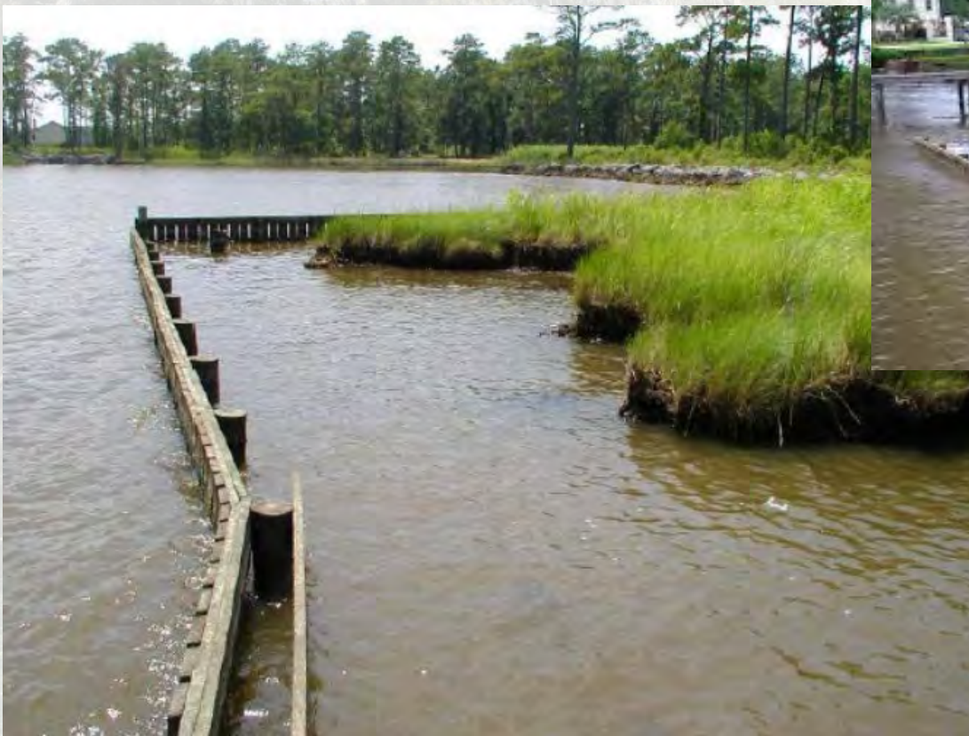
Sheetpile Sill, North Carolina
