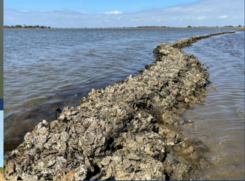
Oyster shell bag breakwater Sweetwater Lake, Galveston TX Photo courtesy of GBF
