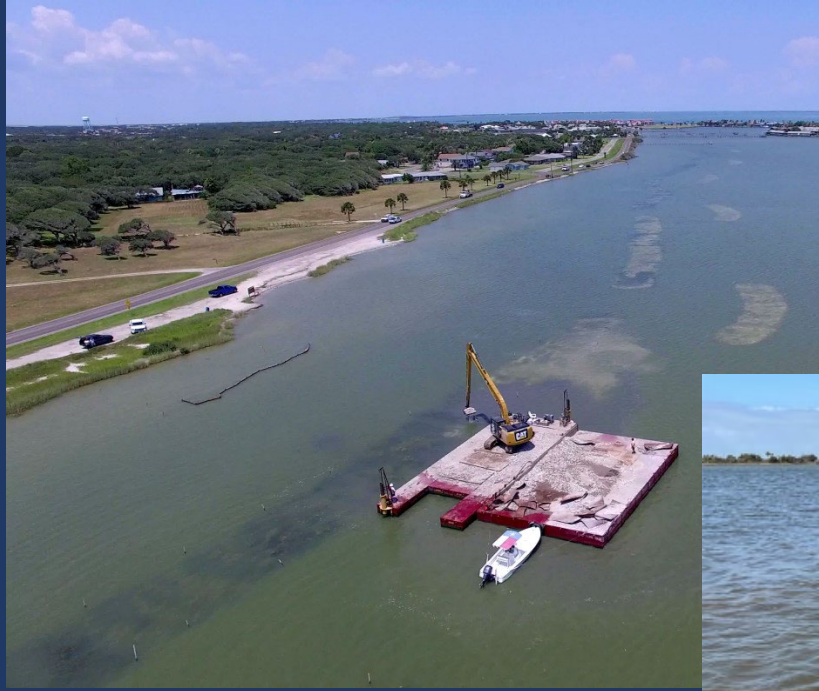
Gabion submerged shell beds Little Bay, Rockport TX Photo courtesy of AECOMv
