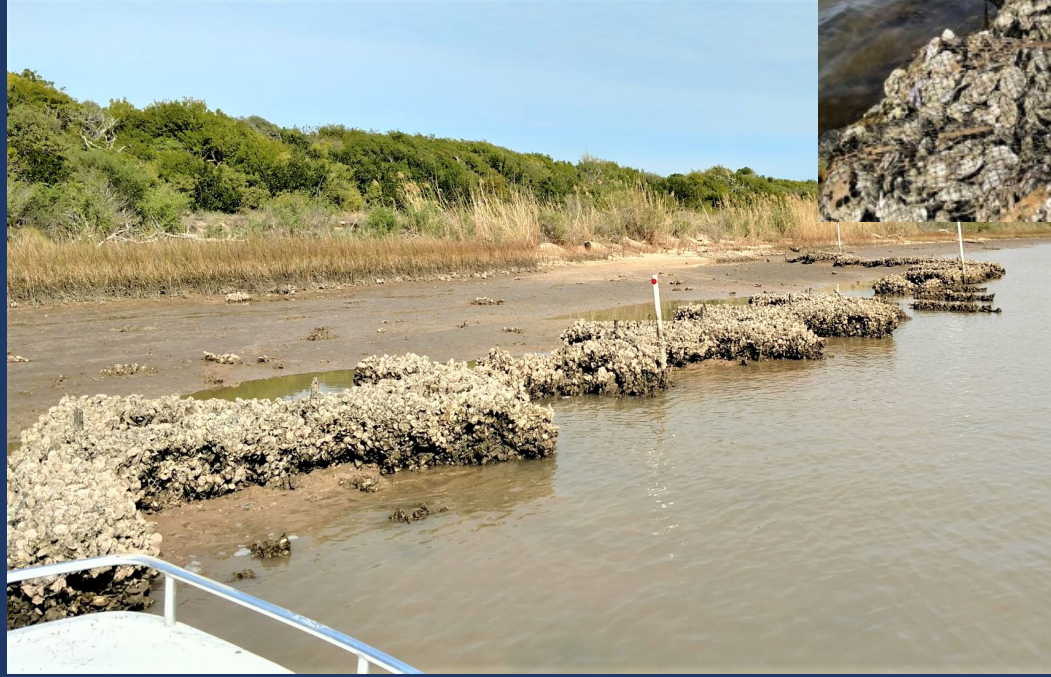
Oyster ReefBLK gabion structures Mad Island Marsh Preserve, Matagorda Bay Photo courtesy of D. Buzan
