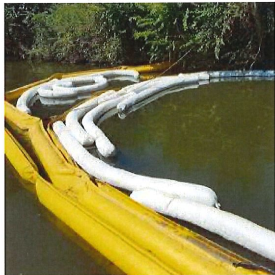
FIGURE 3-3 Containment Booming Strategies after SWA Application
